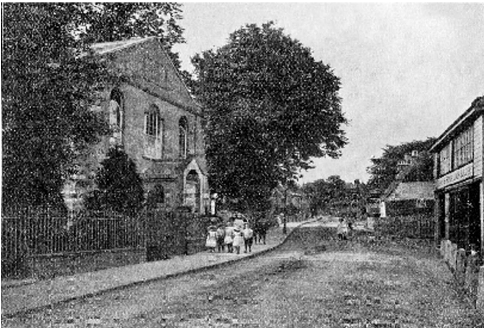
Old photograph of Zion Chapel looking north up Mount Street showing the old porch (now removed). From the frontispiece of Butt-Thompson's book.
